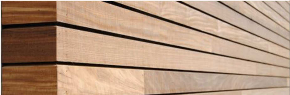
Timber Cladding - with Resene Waterborne Woodsman 'Natural'
